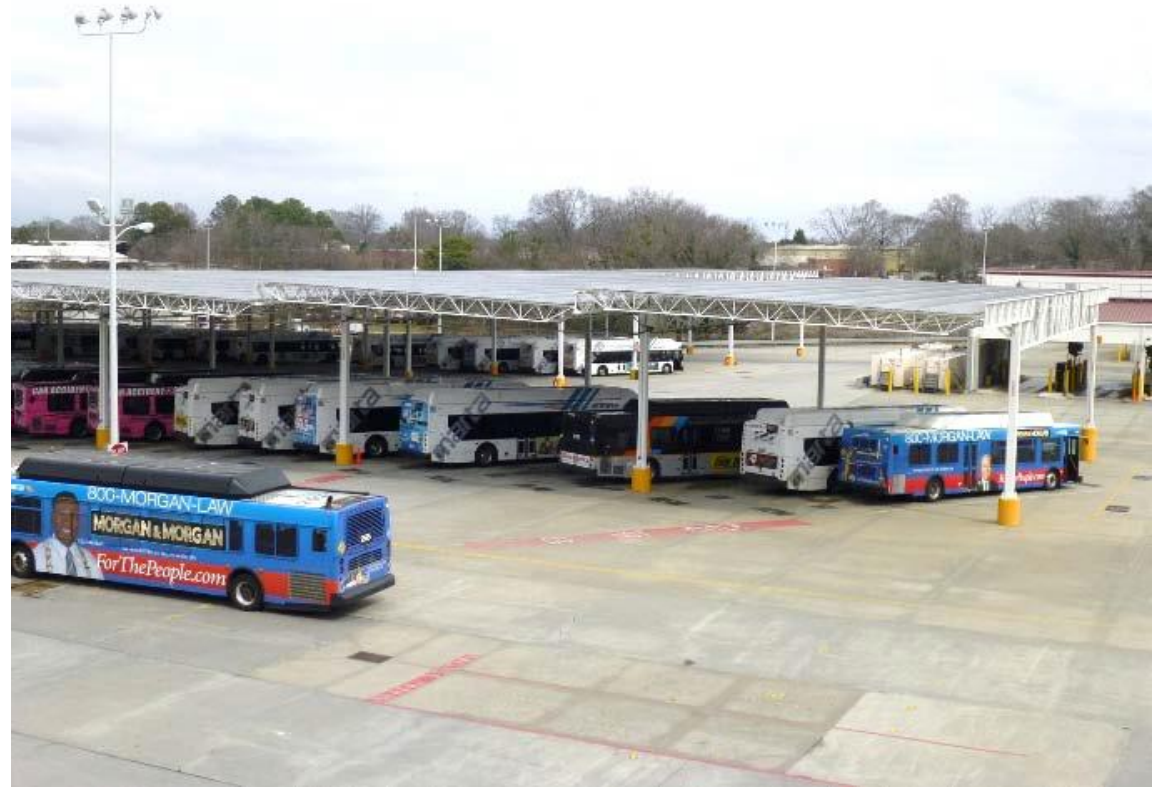
1,200 kW solar canopy at Laredo Bus Facility
